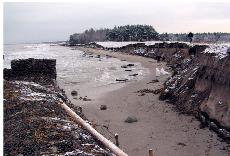
Coastal erosion outlined after storm surge (2018, LSM)
